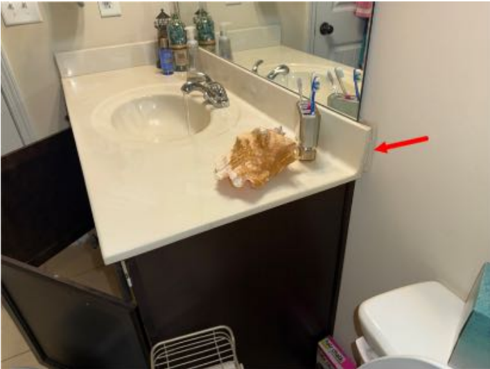
Countertop moves freely. Resecuring recommended.
