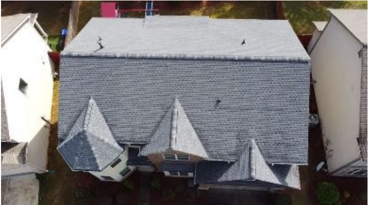
Roof Overview. No major deficiencies noted at shingles, ridge or vent boots at time of inspection.
