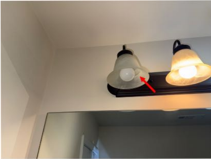
Light not functional. Check fixture with bulb to ensure function.
