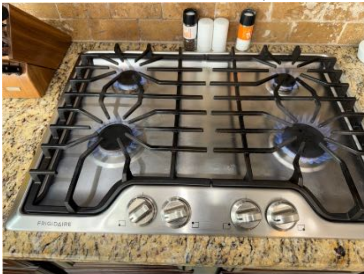
Range functional at time of inspection.
