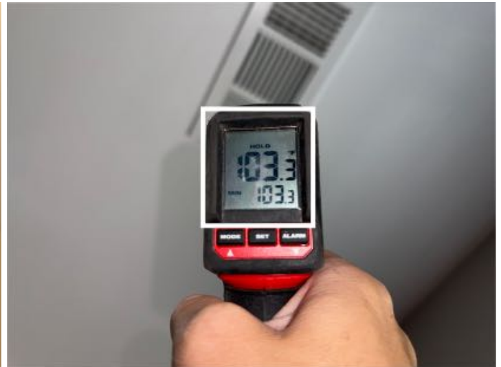
Main level heat tested good at 103 Deg
