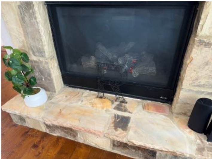
Fireplace functional at time of inspection.
